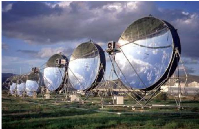
Figure 4: Parabolic Sun Collectors (DLR)
