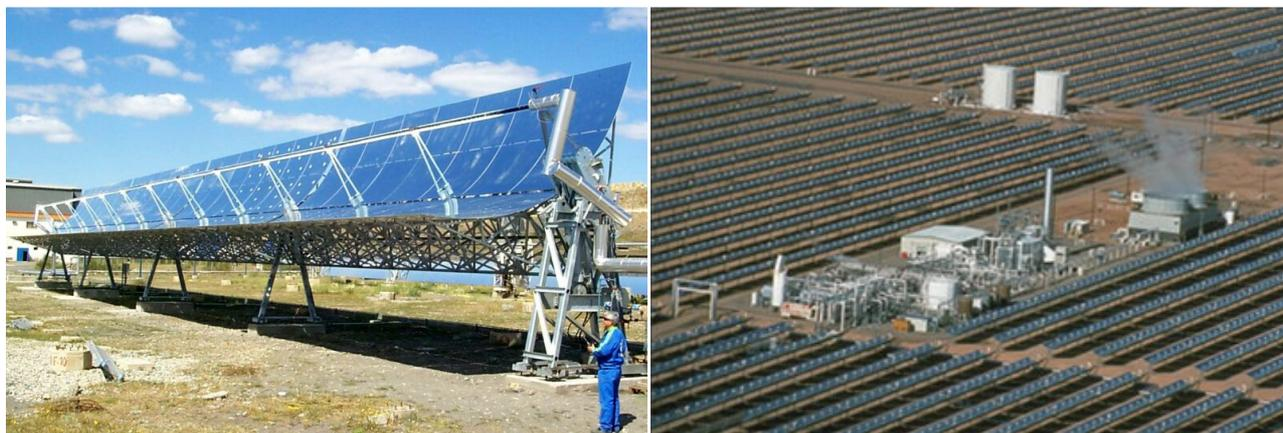
*Figure 6: Parabolic Trough Solar Collectors*
